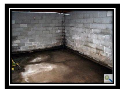
White, flaky powder coating concrete walls and floors is caused by a naturally-occurring mineral salt called "efflorescence". This is a powder that's left behind as water vapour passes through the concrete walls and floors. Over time, these mineral deposits build up in layers so thick that it's sometimes mistaken for mould.
