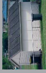
Old Garage: with asbestos cement walls and roof.
