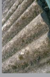
Very poor surfaces of corrugated asbestos cement roof with asbestos debris loose on the roof and in the gutter.
