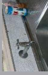
Laminated asbestos cement sheet splash back panel to a sink.
