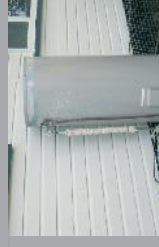
Asbestos woven rope still on a section of hot water pipe leading to a new hot water service unit.
