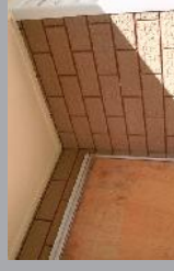
Simulated brick asbestos cement sheet cladding – moulded slices of brick attached to asbestos cement sheeting.
