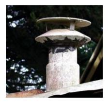
It is very difficult to identify the presence of asbestos just by looking at it. As a general rule, certain building materials installed before the late 1980s may contain asbestos. However, the only way to be certain is to have a sample of the material analysed by a laboratory.
