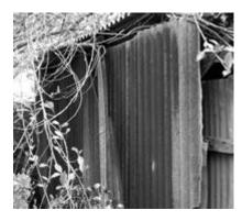
Bonded asbestos materials contain a percentage of asbestos fibres embedded in a hardened cement matrix and are the most common asbestos materials used in residential housing. These materials are commonly called 'fibro', 'asbestos cement' or 'AC sheeting' and can contain 10-15% of asbestos but this figure can sometimes reach up to 40%. <sup>[6]</sup> Today, cellulose fibres have replaced asbestos in fibre cement products.
