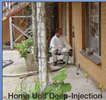
Uretek resin aggressively seeks out voids and fissures, filling them, compressing weak zones.
